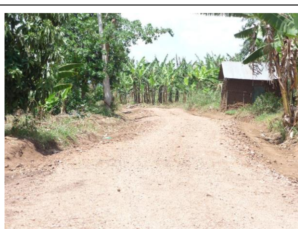
FIGURE 6: FEEDER ROAD UNDER CONSTRUCTION
