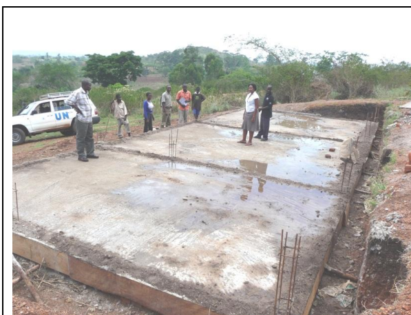
FIGURE 5: SCP UNDER CONSTRUCTION IN KAMWENGE
