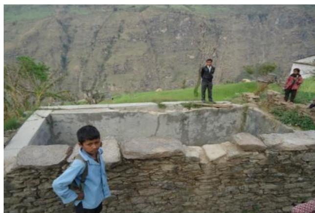
The irrigation pond at Gauterkhal which is cracked and not functional. The potential benefits of this asset are significant, however, no maintenance mechanism is in place.
