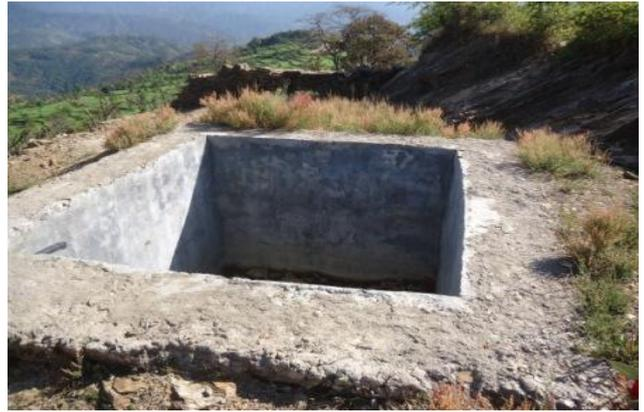
The drinking water tank at Gunpal is not functional as there was no supporting infrastructure provided with the pond. Therefore water cannot be distributed to the houses where it is needed.
