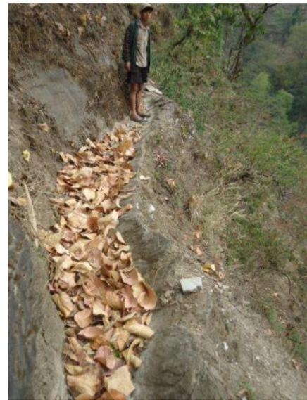
The irrigation channel where it has been cut into the rock.
