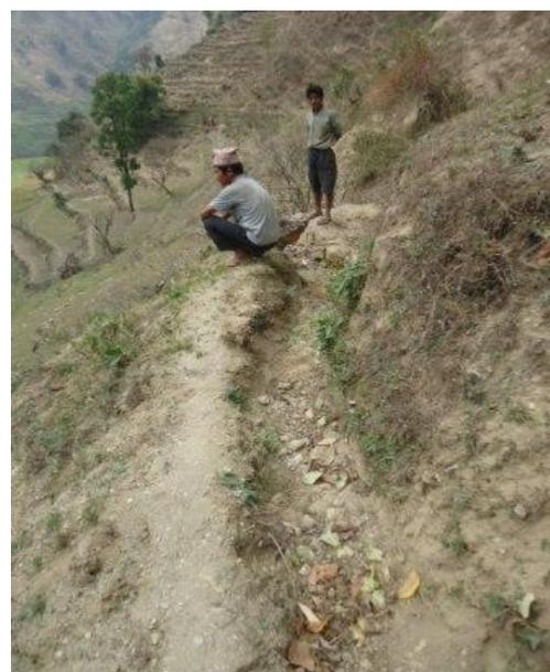
The irrigation channel is mainly earthen in its construction and is reported to still be functional.
