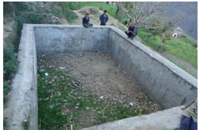
The irrigation pond at Gautarkhal is not functional due to cracks in the cement which causes leakage. No maintenance mechanism is in place to keep the pond in working order.
