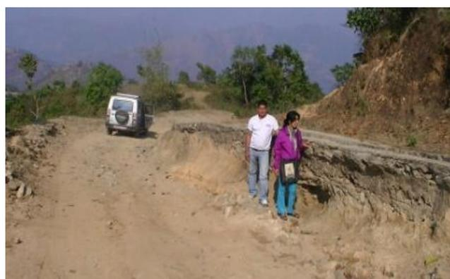
Lack of provision for proper maintenance has left its toll on many sections of road with erosion causing much damage. Here the drainage channel built alongside the road is now above the level of the road it was built to drain water from.
