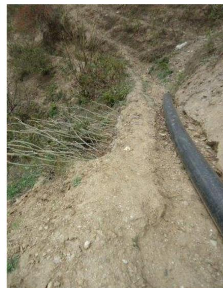
The irrigation channel where plastic pipe has been used to carry the water.
