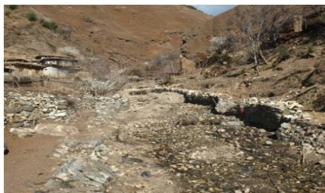
The river embankment strengthening with gabion boxes. This method worked well for some years, reducing the occurrence of flooding. However, lack of maintenance means the threat of flooding has returned as this asset ceases to be functional.
