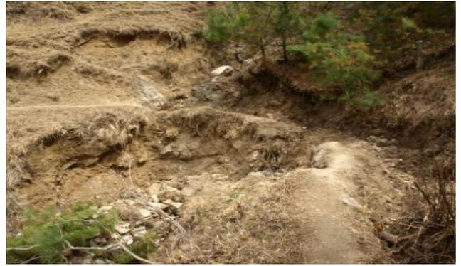
An irrigation channel at Chulakot has several sections where landslips have broken and/or blocked the flow of water. Benefits from this irrigation channel are drastically reduced as a result.
