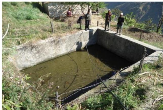
The irrigation pond at Deupatal which is the only pond asset in the VDC to function at all. Most have cracks in the cement and leak.
