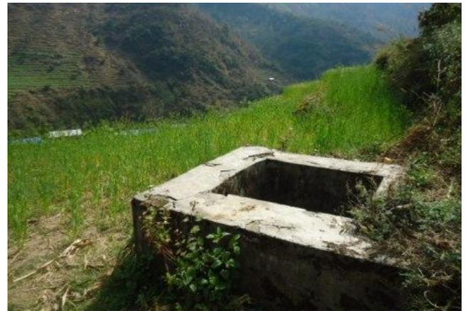
The irrigation water storage tank is an above-ground cement structure and feeds the irrigation system for surrounding land.
