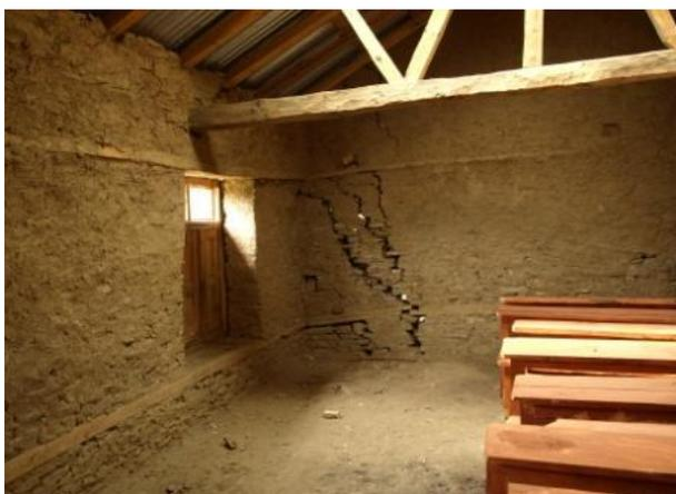
The wall of a school building at Chulakot has a large crack in it. This building is no longer in use by the school for fear of collapse.
