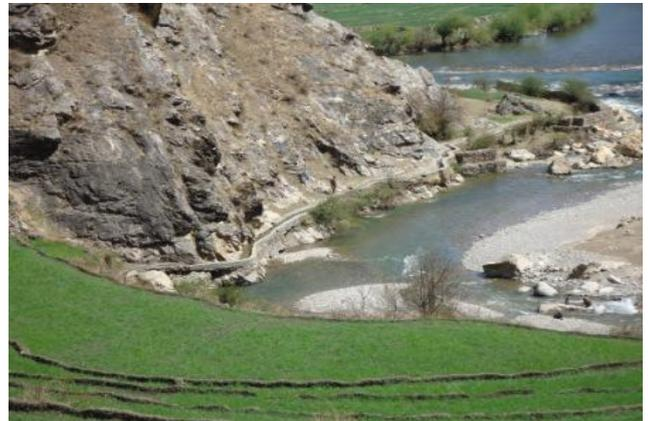
The irrigation channel can be seen along the side of the river. Lack of proper maintenance has left sections in poor condition reducing the benefits to the community.
