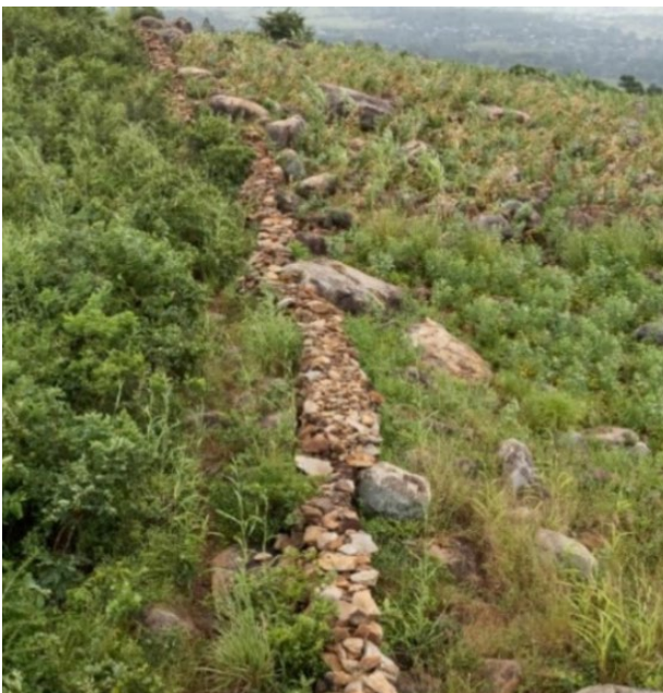
Stone bund under asset creation activities in Phalombe
